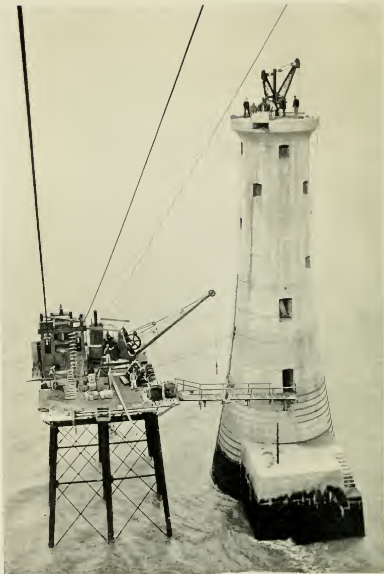
SETTING THE LAST STONE OF THE BEACHY HEAD LIGHTHOUSE.
