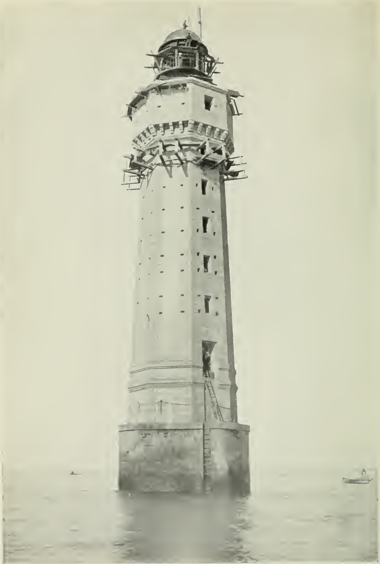
FITTING THE LANTERN OF LA JUMENT LIGHT.
